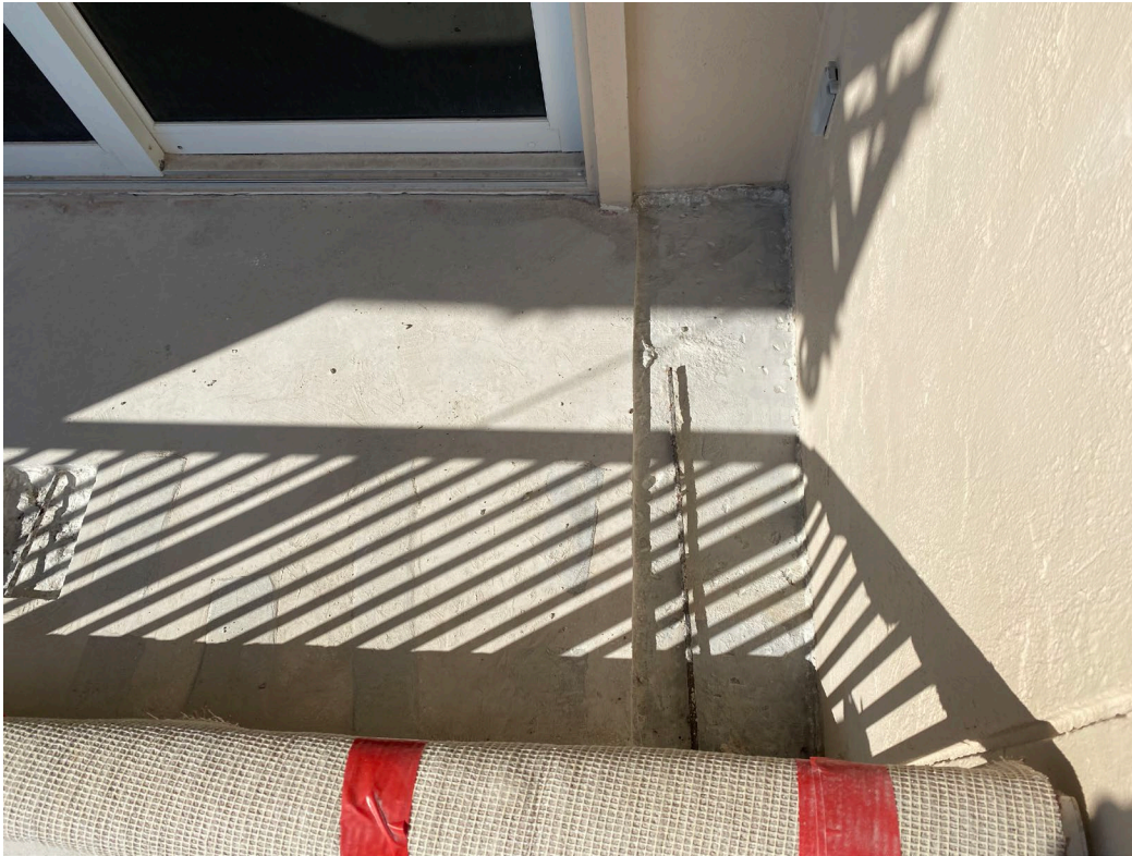
Picture 1: Typical concrete repairs
