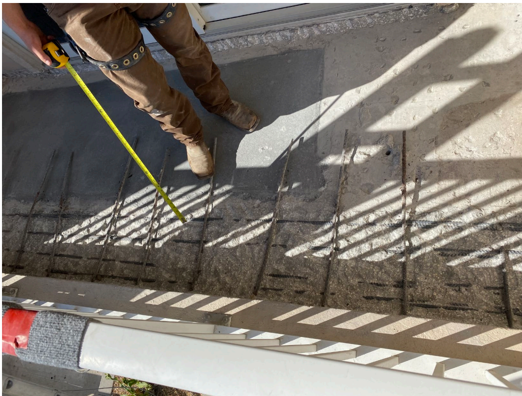
Picture 2: Typical concrete repair
